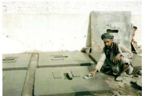
Latrine slab construction - Participatory Integrated Development Society
