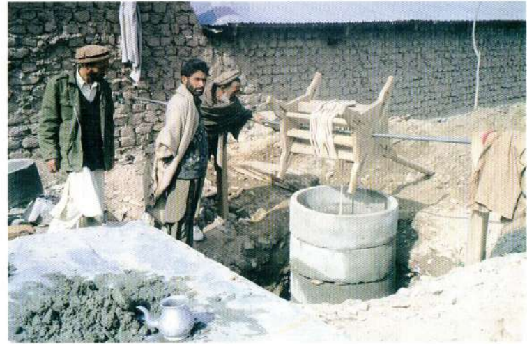
Hand pump construction - Participatory Integrated Development Society
